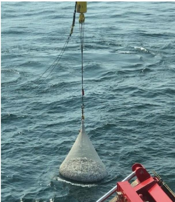
Loose rock placement can be achieved using a flexible fall pipe to deliver rock to the seabed in a controlled manner. The rock cannot be removed as easily after deployment but is more efficient for larger areas than numerous rock bags. Rock berms with tapered gradients can be made so that they are trawlable, but this can extend the volume and area of rock required. Rock placement in this manner is the most common method of scour protection around OWF foundations.
